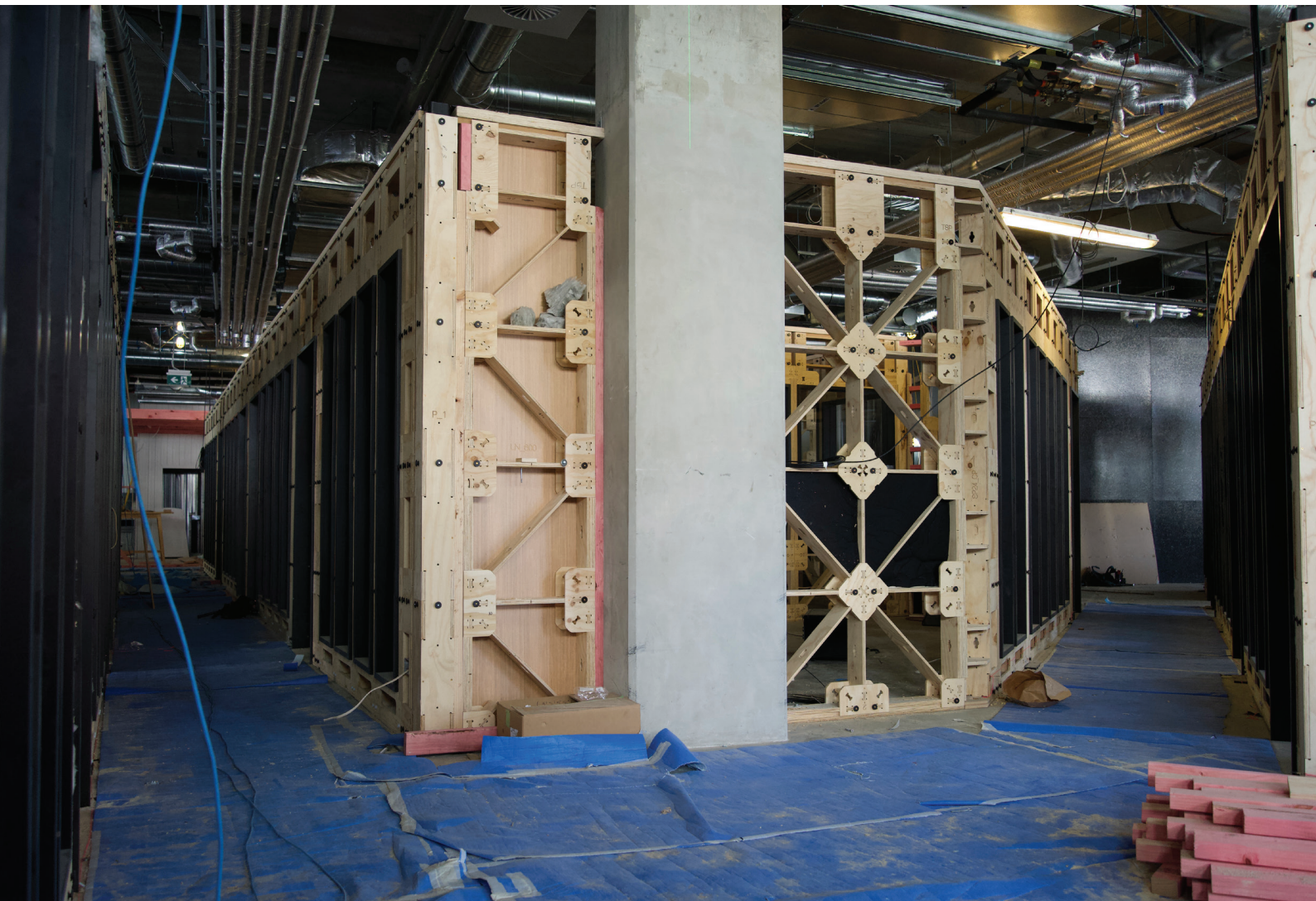
Installation of XFrame Walls and Windows
